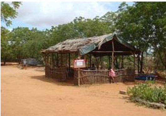
Tukul at CFS in Ifo Section N where SC Complaints Desk is Located.
