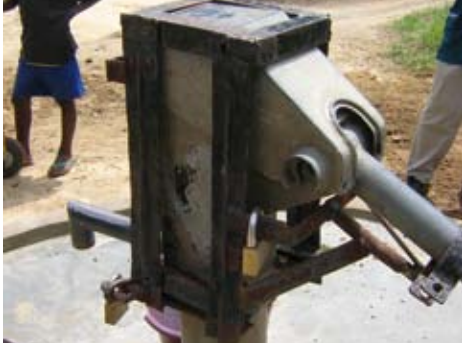
Metal 'jacket' placed over the top of a hand-pump by the community water committee in the Chicken Soup Factory community in an urban area in Monrovia, Liberia to prevent theft and use without payment
