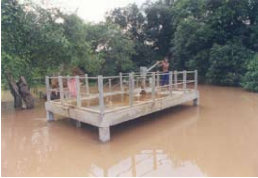
Ro'Ang Leu flood (2001) – raised handpump with platform
