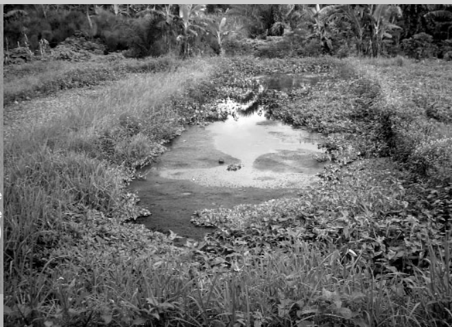
Station de lagunage de Biyenassi, Yaoundé (Cameroun)
